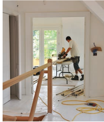
The house is abuzz with saws and drills as the construction crew and tradesmen move indoors to build the banisters, finish the trim and fit our custom pieces.
